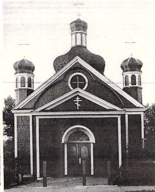
Figure 4. Holy Ghost Ukrainian Greek Catholic Church, before 1978 renovations. Photo courtesy of the Beaton Institute.
